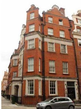
View from the corner of Mount Street and Balfour
