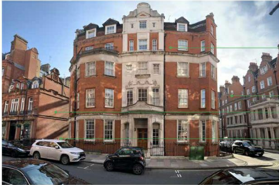
North elevation of No.82 Mount Street and 6 Balfour Place
